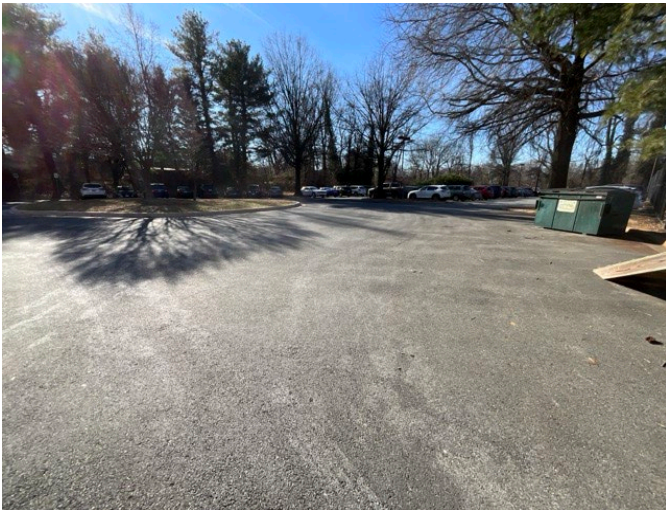
33 - REAR PARKING LOT
