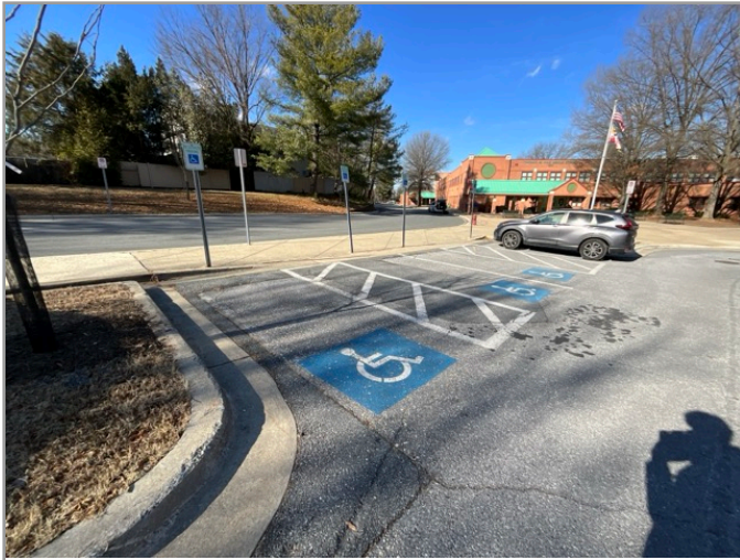
OVERVIEW OF ACCESSIBLE PARKING AREA
